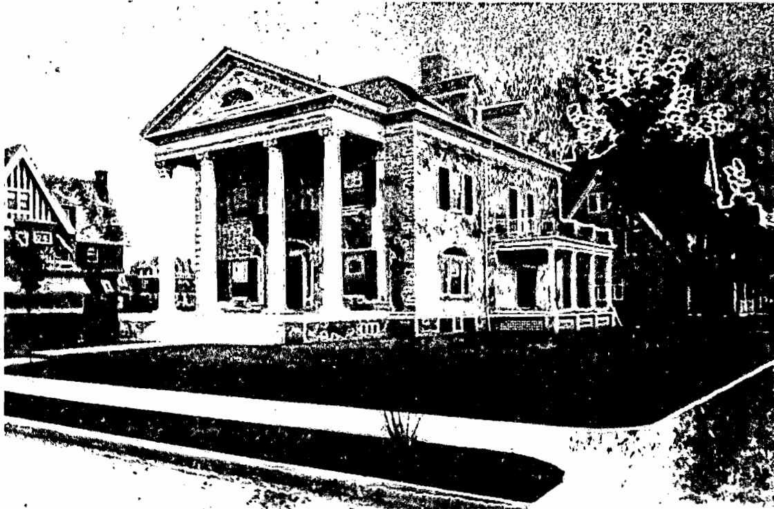
1510 Albemarle Road. John J. Petit, 1900 (From Architects' and Builders' Magazine , January, 1902).
