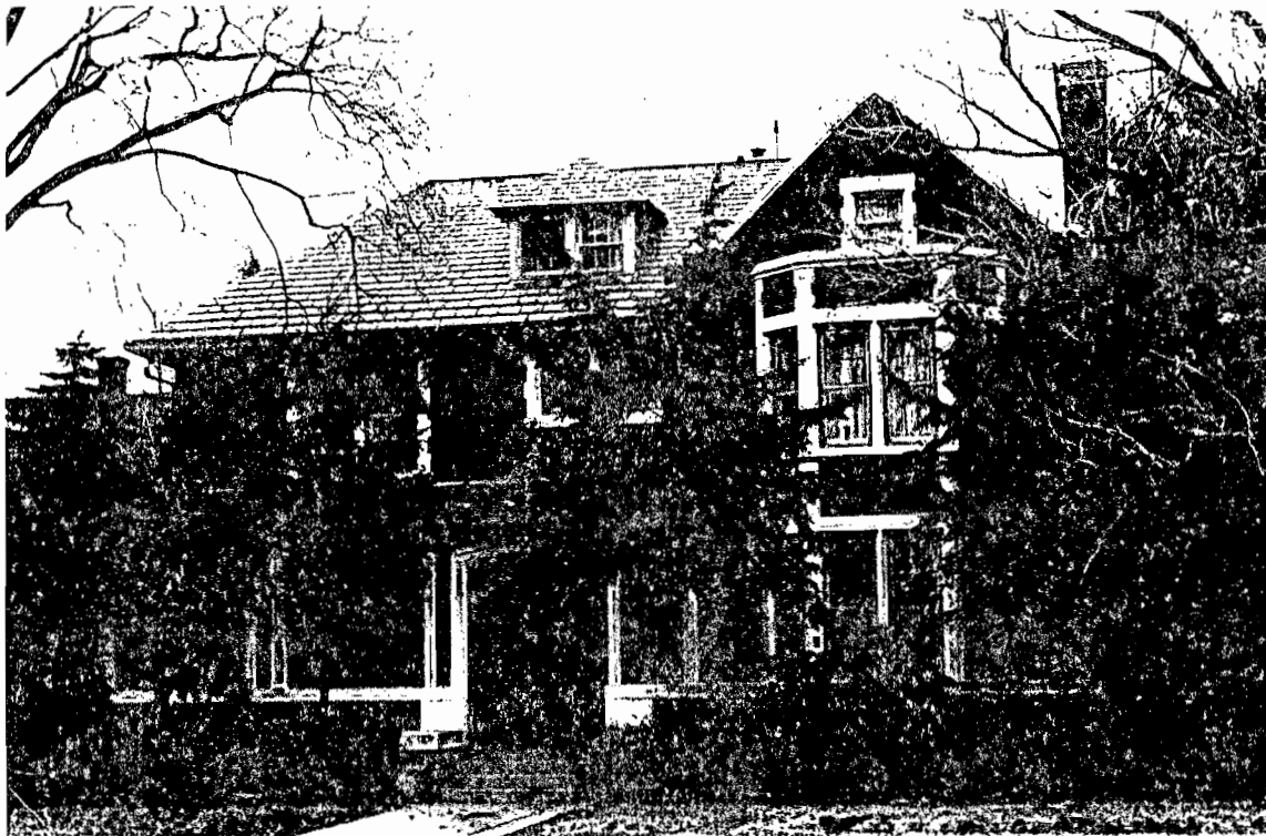
1325 Albemarle Road. Architect unknown, c. 1912.
