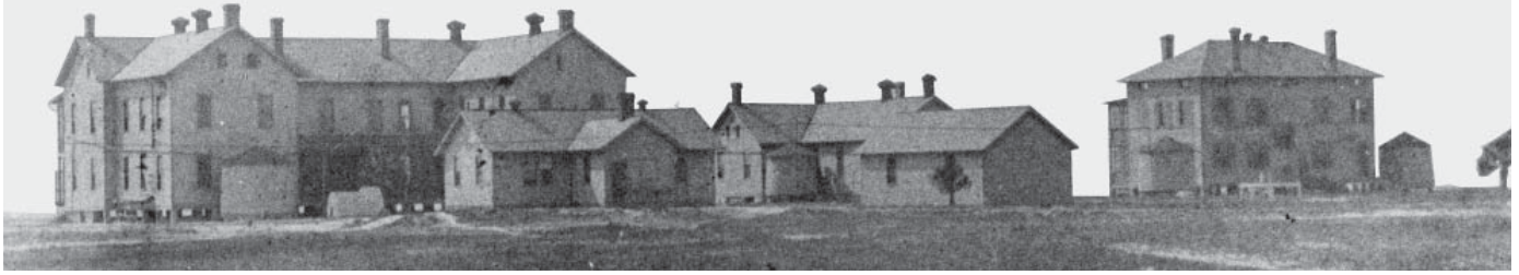
Fort De Soto Buildings
